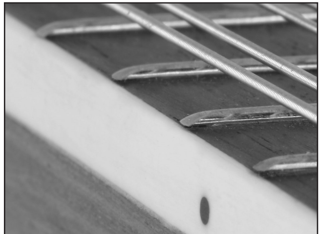
Figure 30. Example of correctly angled fret ends.
